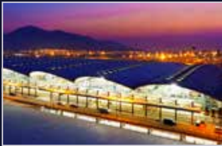
Hong Kong International Airport
